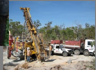
Drilling at Kingsgate
