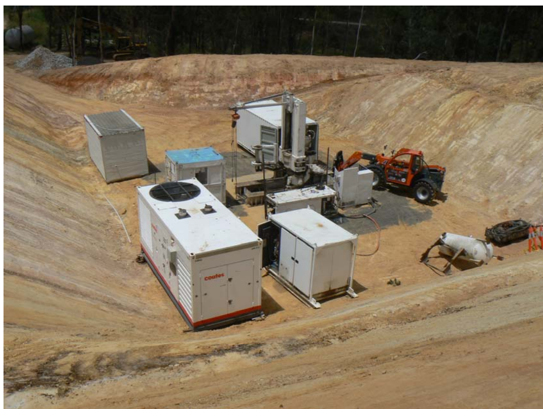
Raise bore equipment at Exhibition for 2.4m shaft
