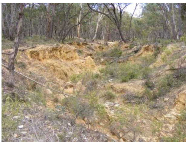
Erosion area January 2008.
