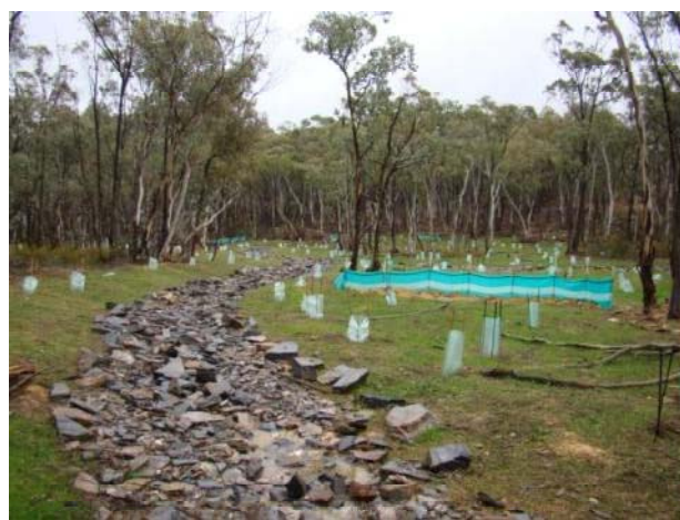
Completed rehabilitation June 2008.
