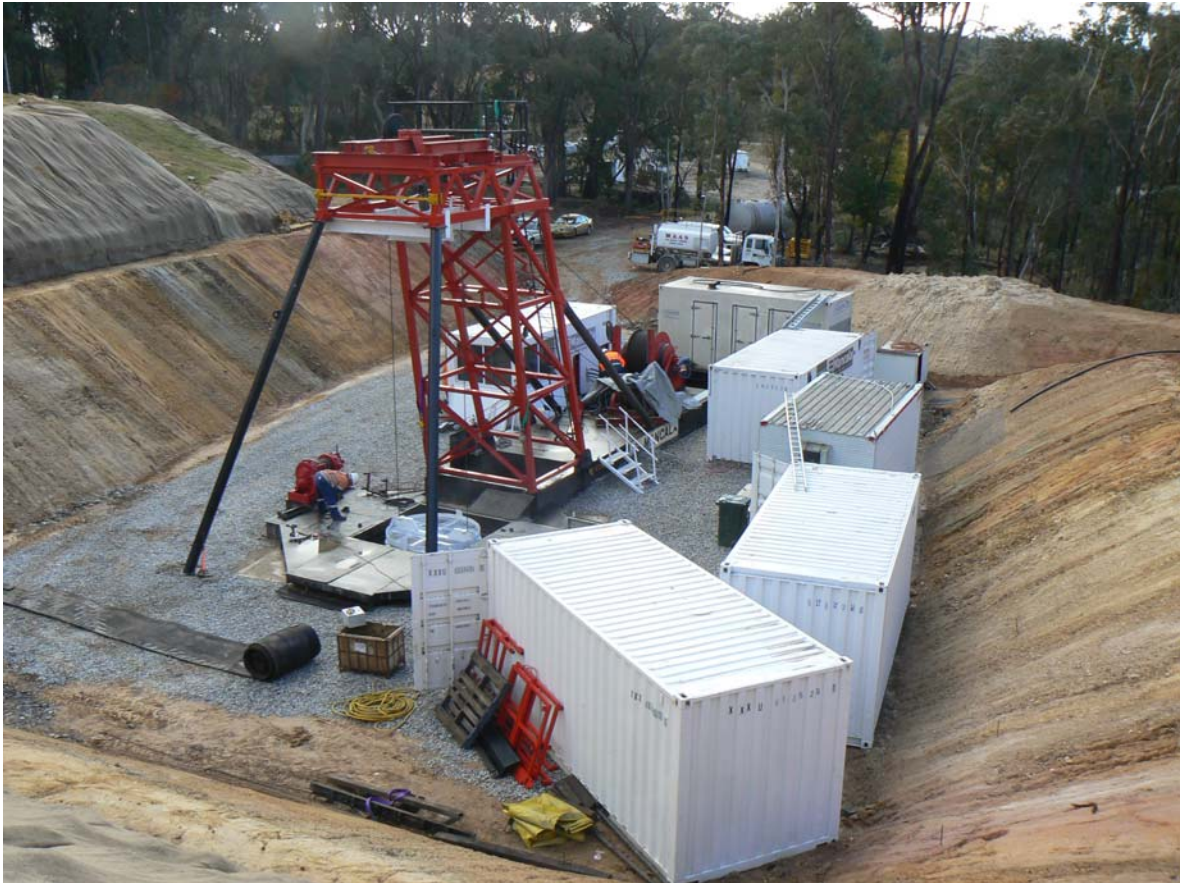
EQUIPPING HEADFRAME AND STAGE OVER RAISE BORE SHAFT
