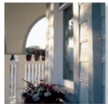
Door and Window Surrounds
