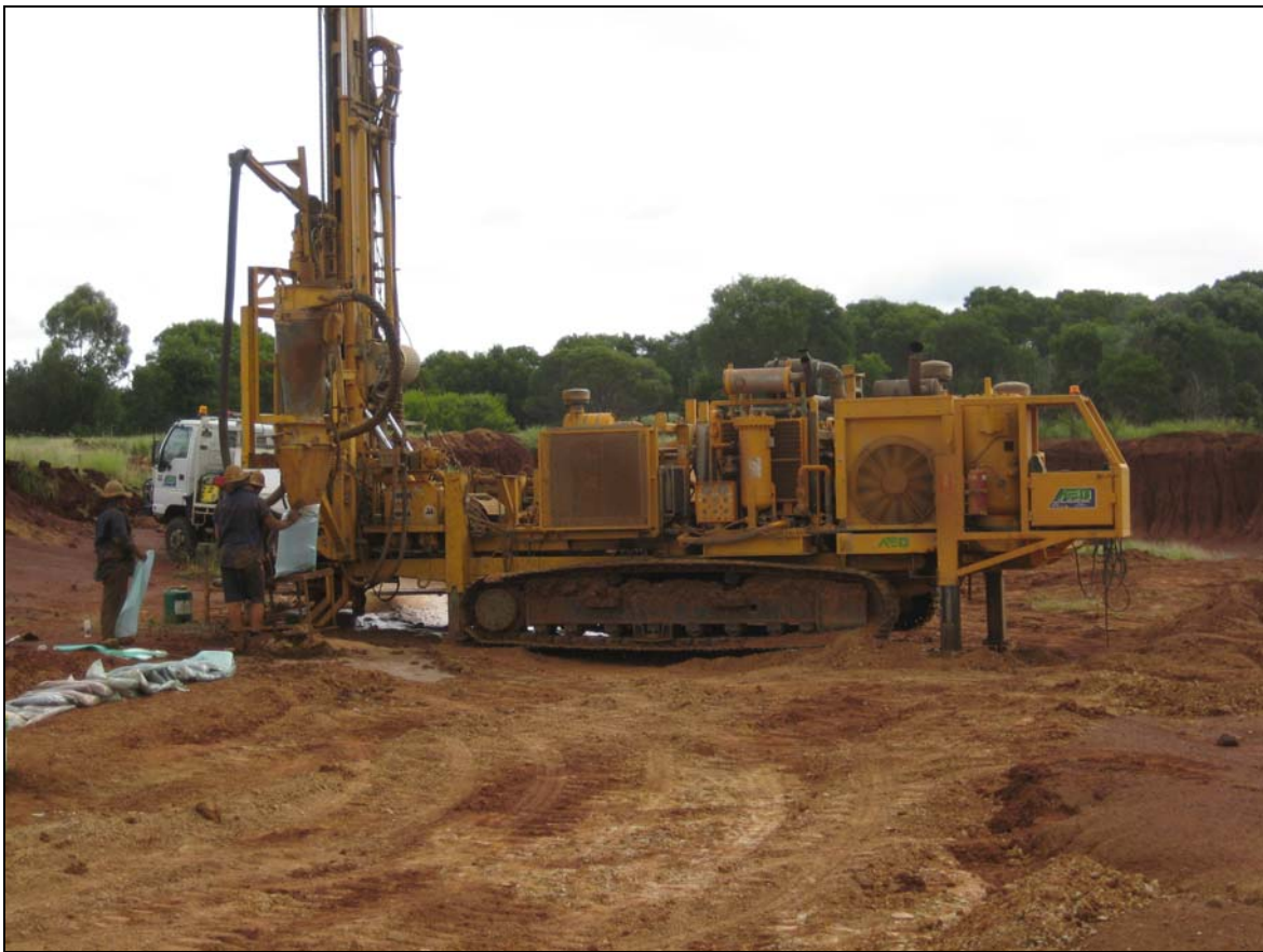
RC Drilling at the Edge – Greenvale Mine Site
