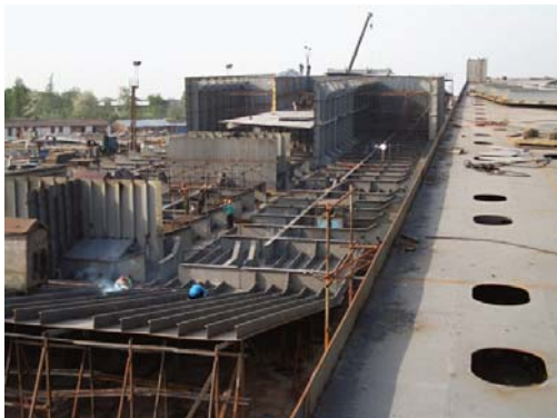
Barge Under Construction
