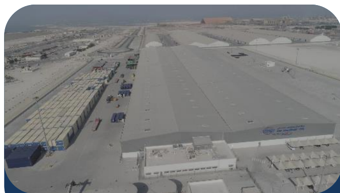
CSP Abu Dhabi CFS Phase 1
