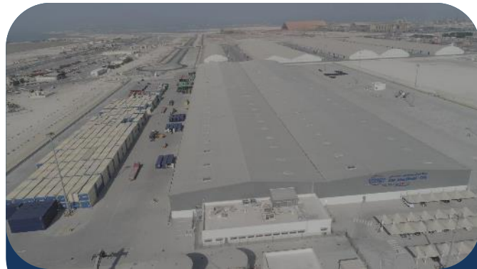
CSP Abu Dhabi CFS Phase 1
