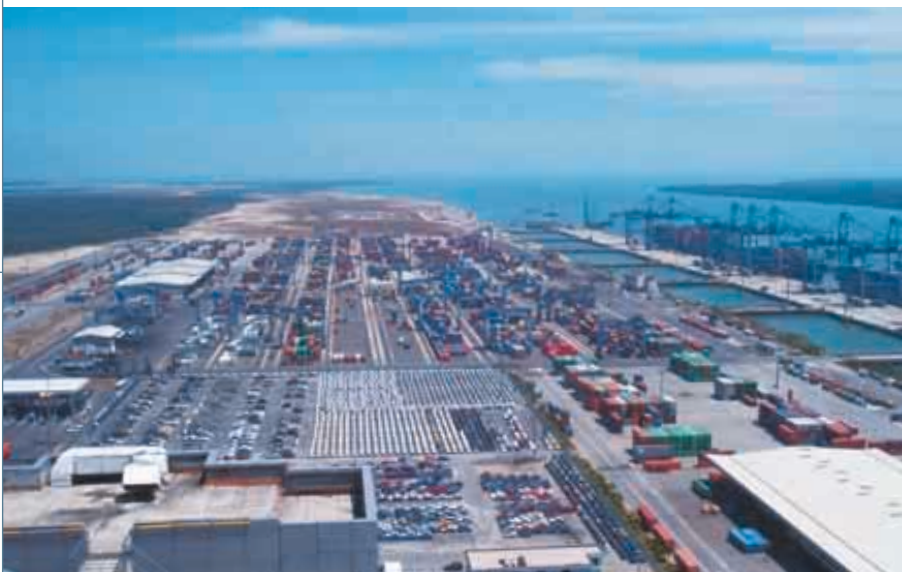
KMT-Westport, Port Klang, is equipped to handle containers, dry bulk, liquid bulk and conventional cargo.
