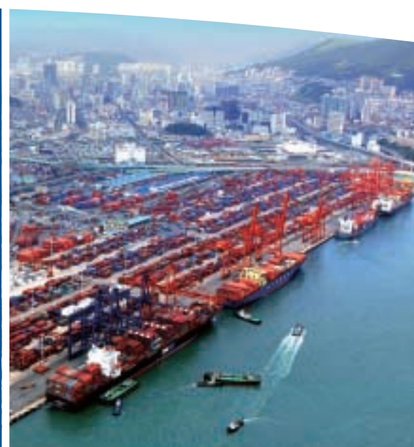
An aerial view of Hutchison Busan Container Terminal.
