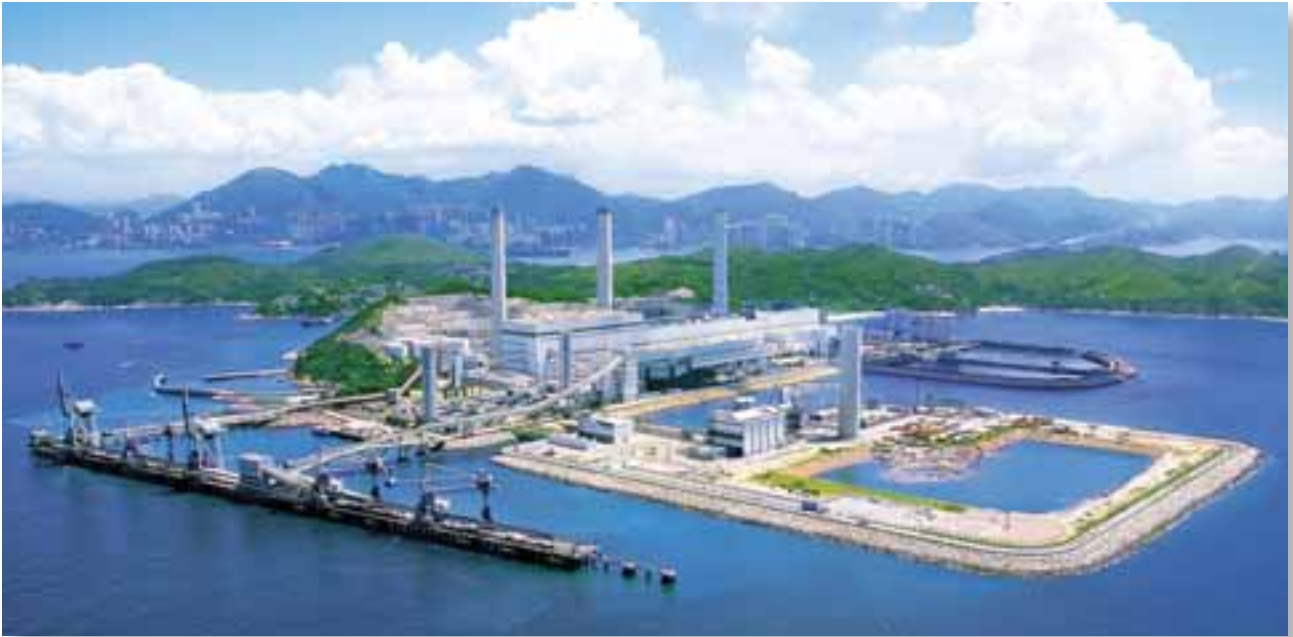
■ HK Electric's Lamma Power Station provides electricity to customers on Hong Kong Island and Lamma Island.
