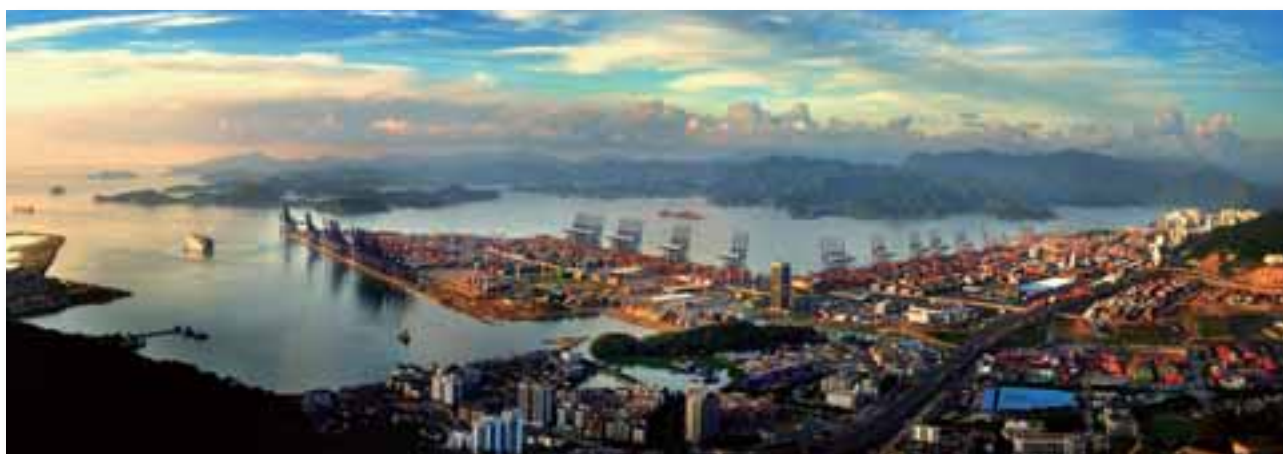
With the completion of the fifth berth at YICT Expansion Project, YICT has a total of 15 deep-water container berths.
