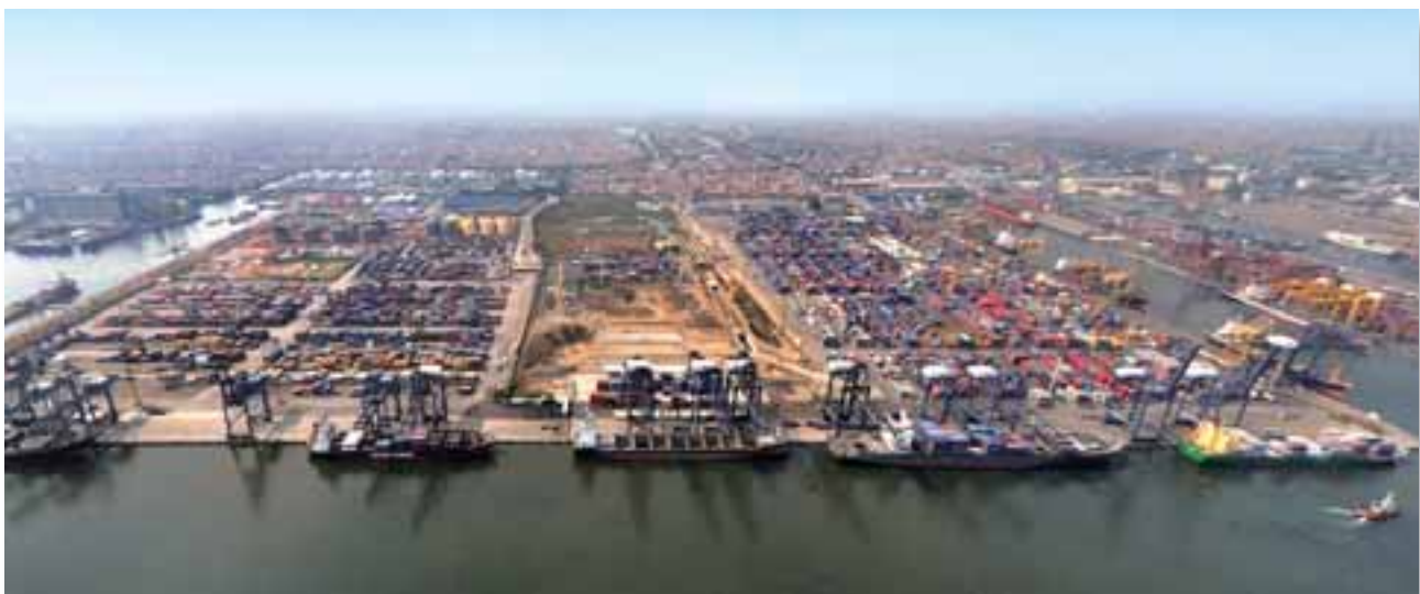
Jakarta International Container Terminal has installed Hutchison Port Holdings' proprietary Next Generation Terminal Management System to enhance operational efficiency.
