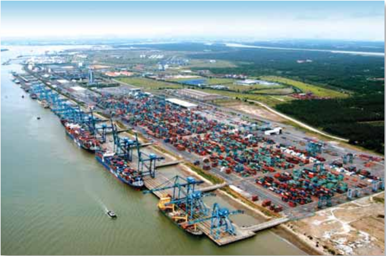
■ An overview of Westports Malaysia.
