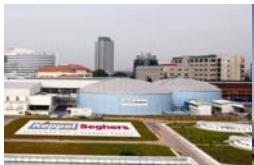
Ulu Pandan NEWater Plant
