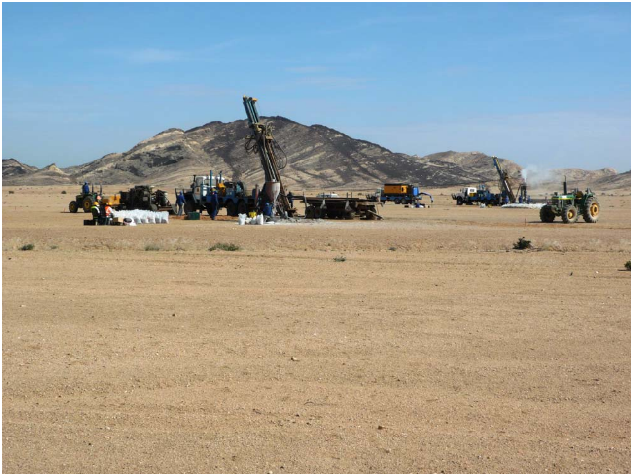
RC Drilling Rigs at the Ongolo Alaskite Project – January 2011
