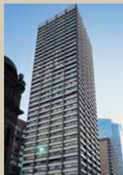
ST MARTINS TOWER 31 MARKET STREET, SYDNEY
