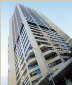
TELSTRA PLAZA (NORTH) 310-322 PITT STREET, SYDNEY
