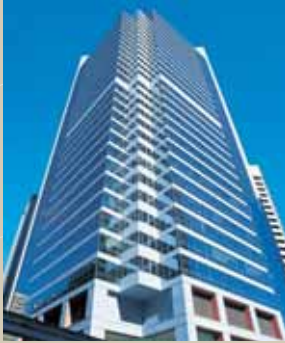
BT TOWER 1 MARKET STREET, SYDNEY
