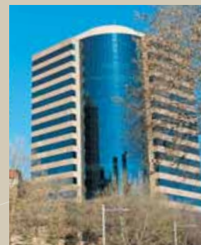
CENTENNIAL PLAZA TOWER C 300 ELIZABETH STREET, SYDNEY
