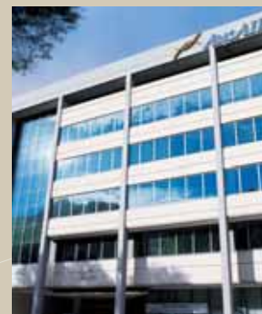
AUSAID BUILDING 62 NORTHBOURNE AVENUE, CANNBERRA
