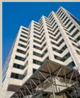
TELSTRA HOUSE 231 ELIZABETH STREET, SYDNEY
