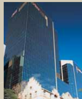
MARITIME TRADE TOWERS 201 KENT STREET, SYDNEY
