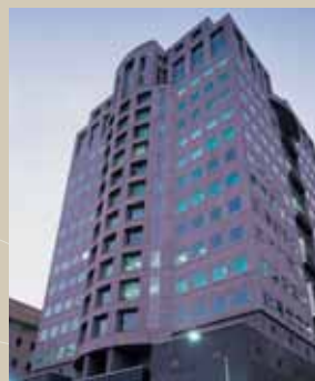
CUSTOMS HOUSE 414 LA TROBE STREET, MELBOURNE
