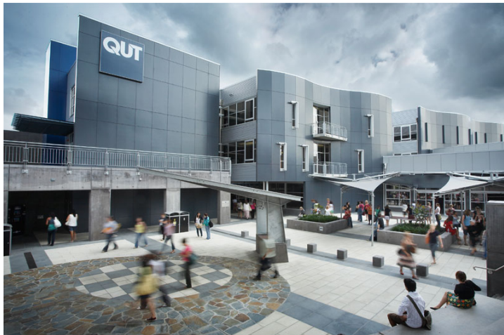
James Hardie ExoTec® Facade Panel and fixing system has been used on the Queensland University of Technology. Architect: Conrad & Gargett.
