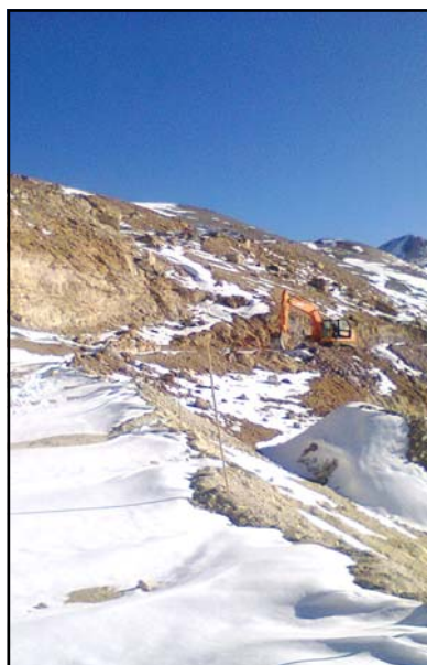
Nueva Esperanza, Chile, access road construction, winter 2014
