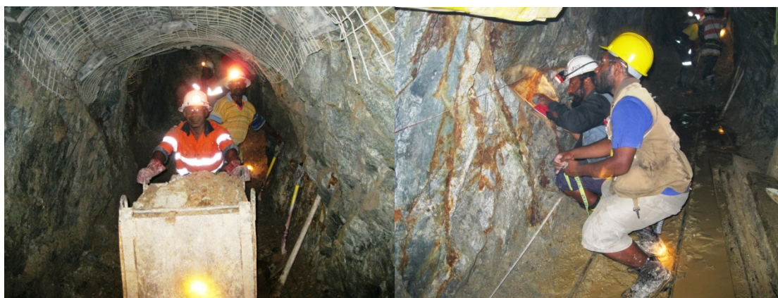
Yandera – Bulk Sample Adit
