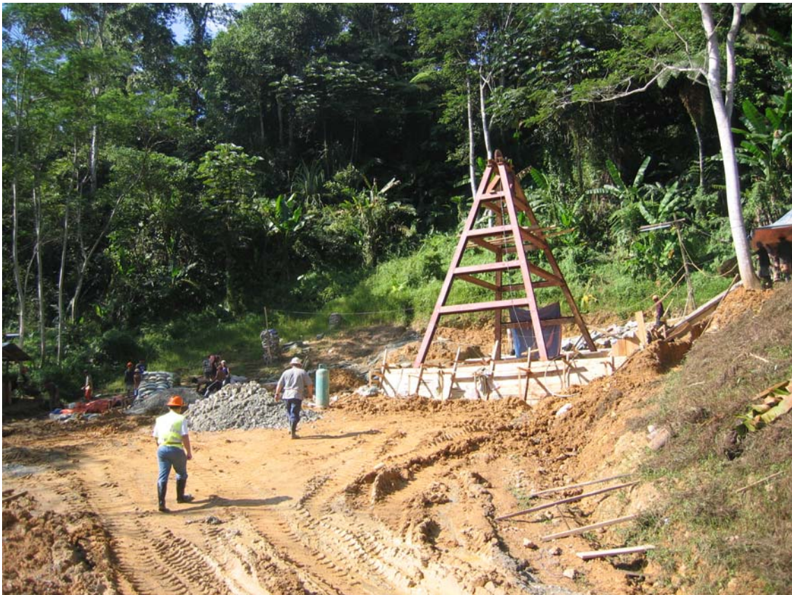
Plate 1. Agsao shaft headframe standing 7.3 metres high.
