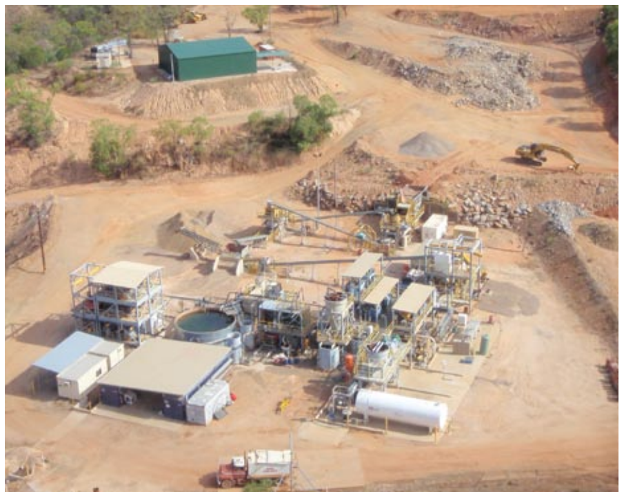
Wolfram Camp Processing Plant
