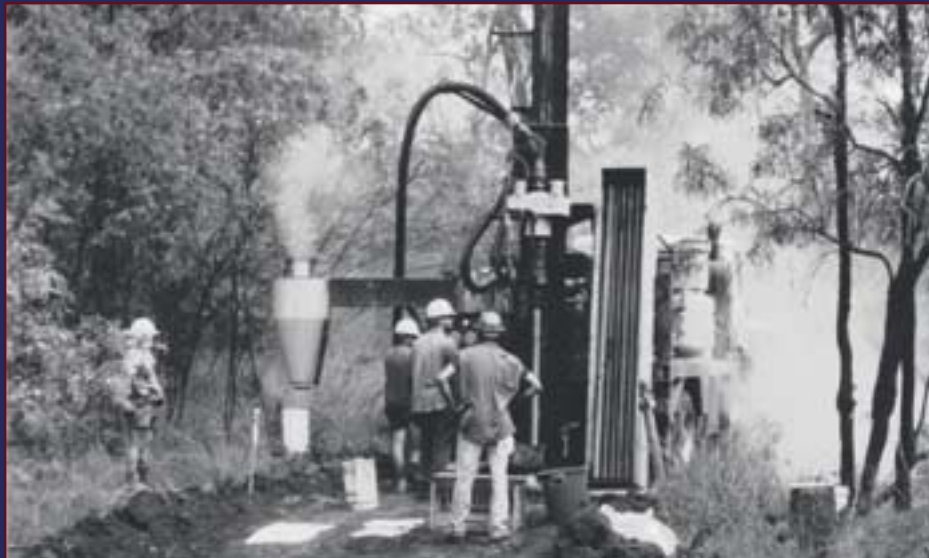
Drilling at Bell Creek Nickel Project – NORNICO
