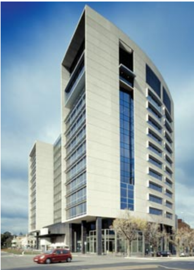
OneSteel recently supplied steel for the 12-storey Law School, part of the University of Melbourne's recent development at University Square in South Carlton. The development consists of three academic buildings and an underground carpark with space for 1,100 cars. The Law Building provides 20,000 square metres of academic and educational space for the University's Law Faculty.
