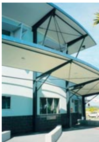
The Varsity College School Complex on Queensland's Gold Coast takes a whole new approach to the design of education buildings, supported by the freedom of OneSteel's products.
