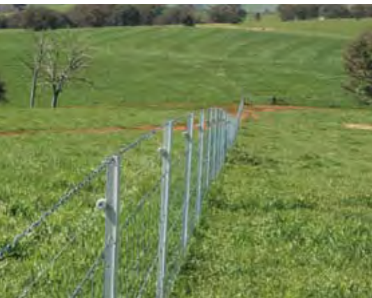
The fence pictured was constructed using Waratah® Stocktite® Longlife™ prefabricated wire, GalStar® fence posts and a single strand of barbed wire.
