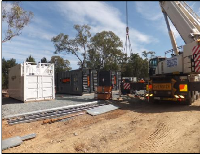
Decline power station installed
