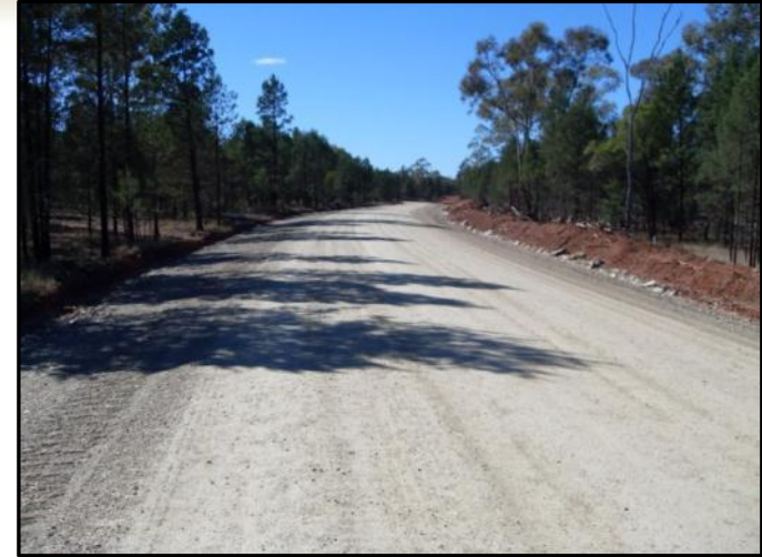
All weather access road complete
