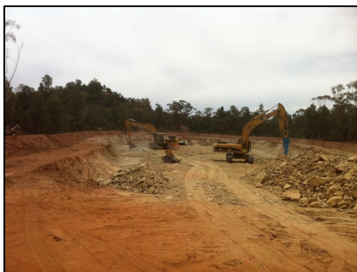
Hera boxcut – under construction
