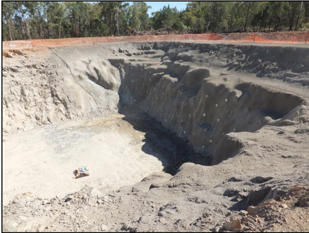
Hera boxcut showing completed ground support on high-wall face
