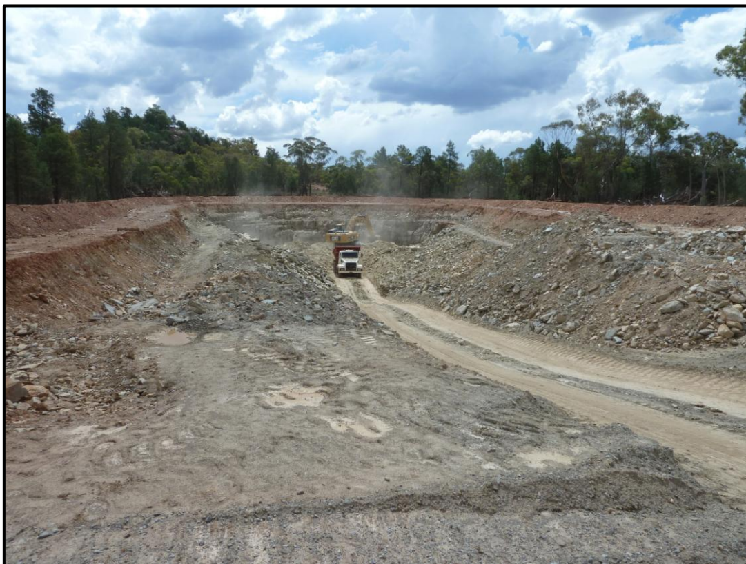
Progress on the Hera Boxcut – February 2012
