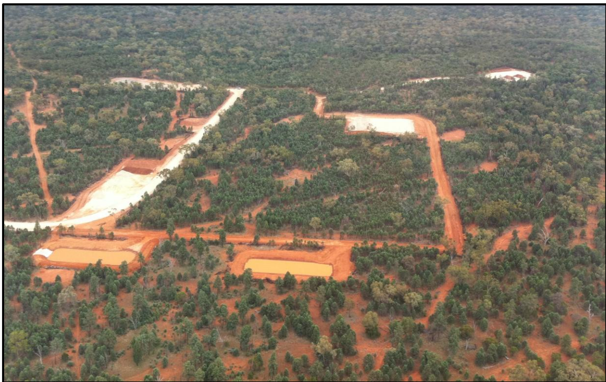
Stage 1 Earthworks completed at Hera – April 2012
