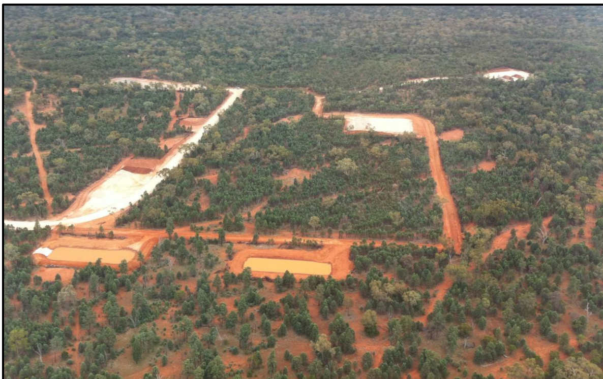
Stage 1 Earthworks completed at Hera – April 2012
