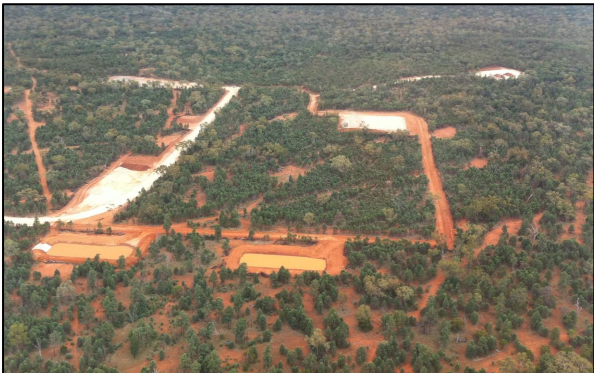
Stage 1 Earthworks completed at Hera – April 2012
