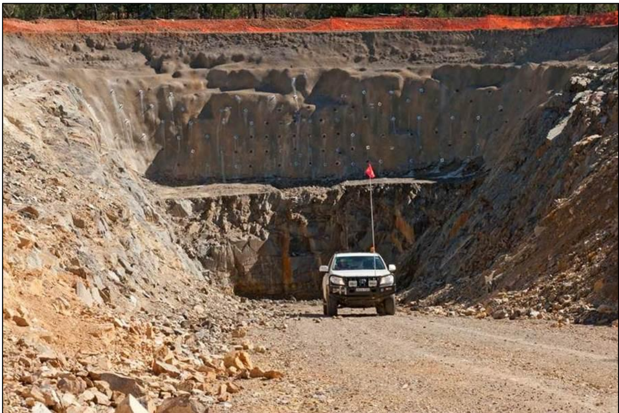
Hera Project – Completed Boxcut
