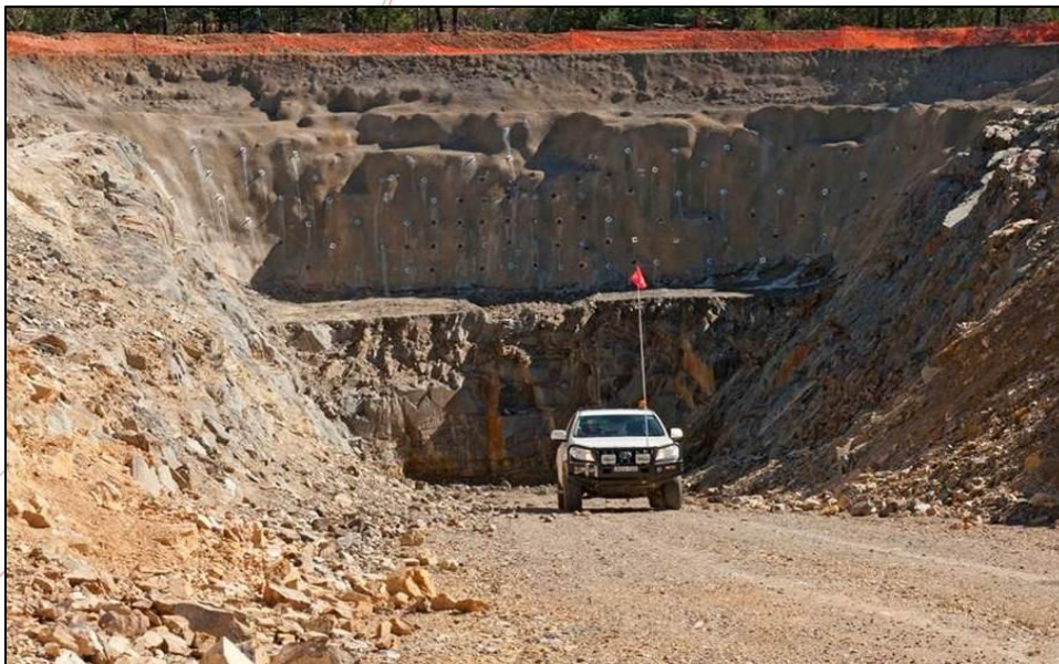
Hera Project – Completed Boxcut
