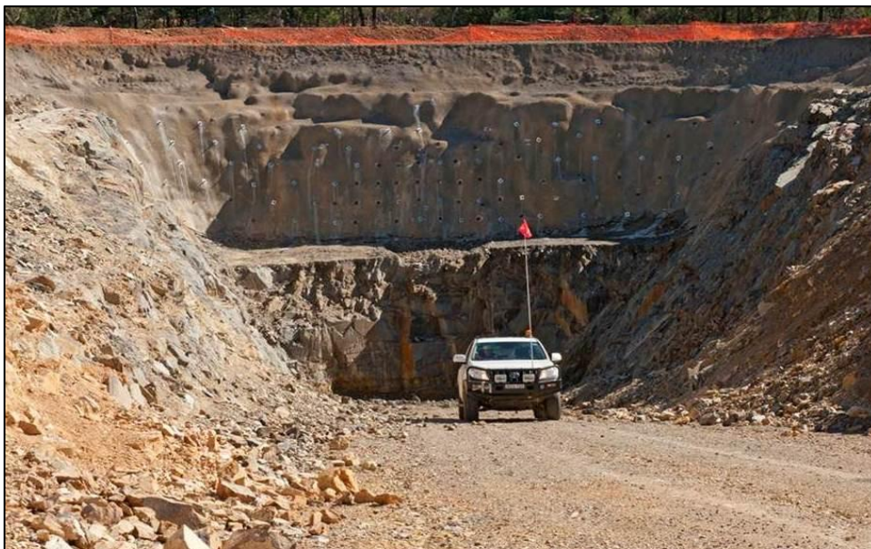
Hera Project – Completed Boxcut
