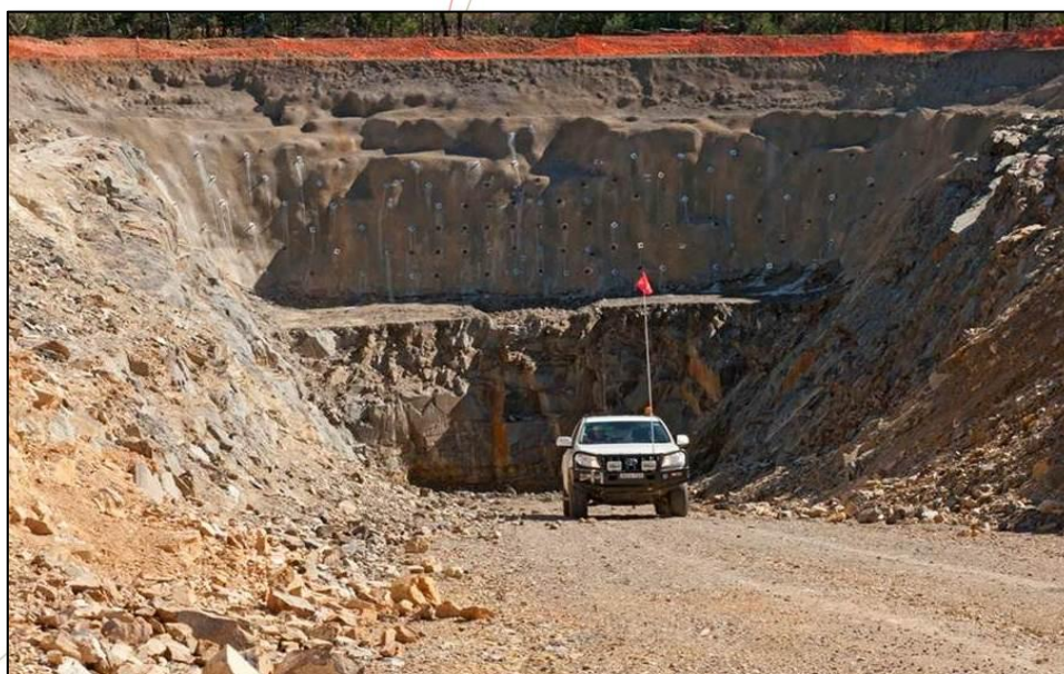
Hera Project – Completed Boxcut
