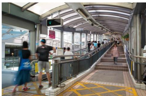
Central-Mid-Levels Escalator and Walkway System, Hong Kong
