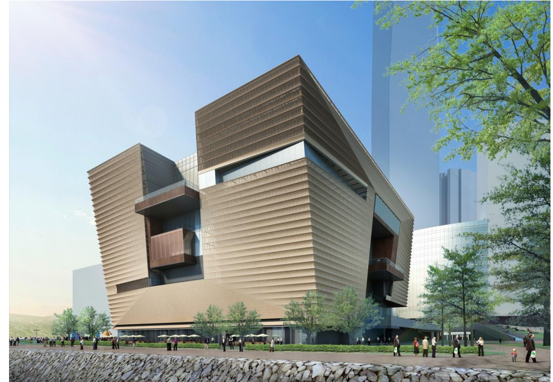
Design, supply and installation of heavy-duty freight lift, Hong Kong Palace Museum Contract sum: HK$ 3.6M
