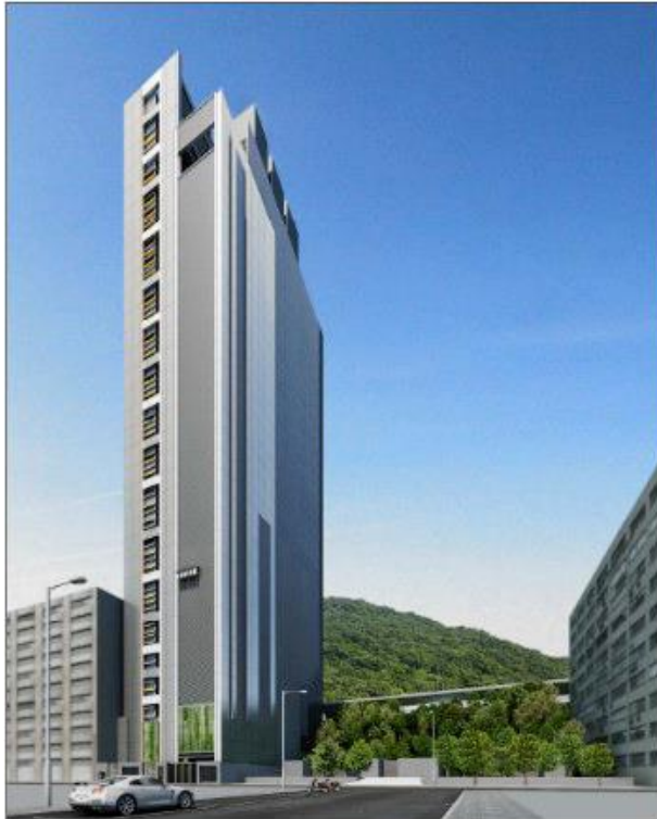
Government Data Centre Complex, Cheung Sha Wan Contract sum: HK$ 900M
