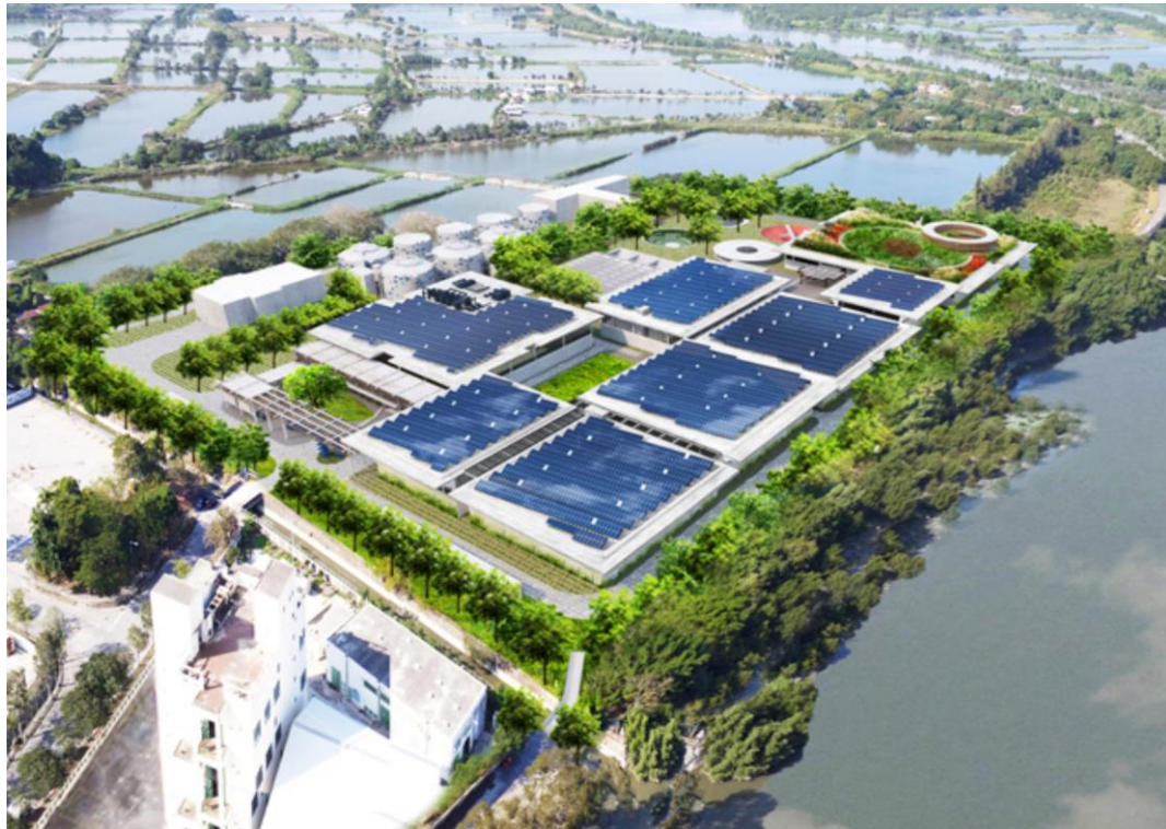
Yuen Long Sewage Treatment Works and Yuen Long Effluent Polishing Plant Contract sum: HK$ 1,228M
