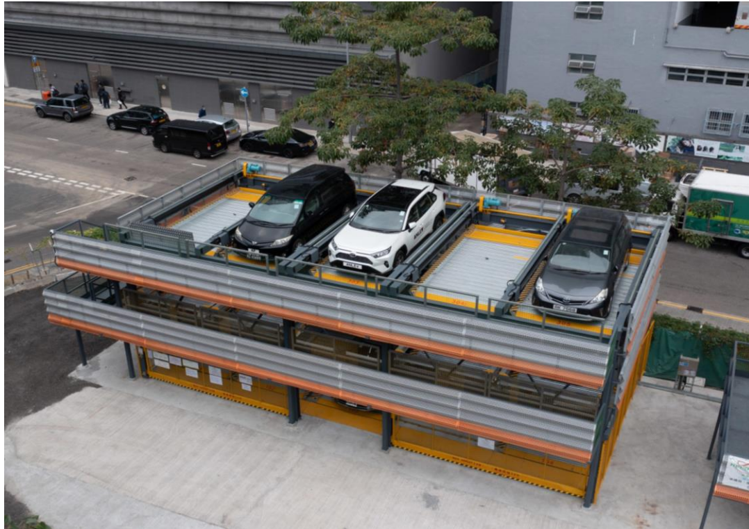
Series projects of Puzzle Stacking Automated Parking System Contract sum: HK$ 7M
