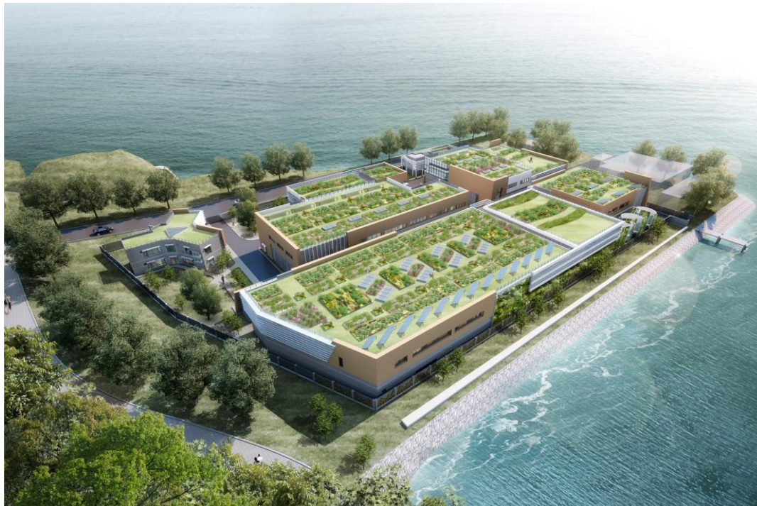
Cheung Chau Sewage Treatment and Disposal Facilities Contract sum: HK$ 306M
