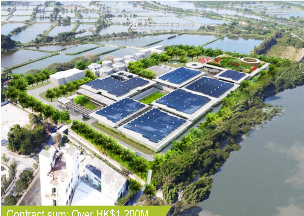
Yuen Long Sewage Treatment Works and Yuen Long Effluent Polishing Plant
