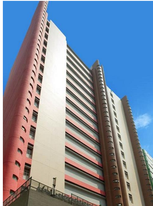
Construction of Data Centre for large local colocation company
