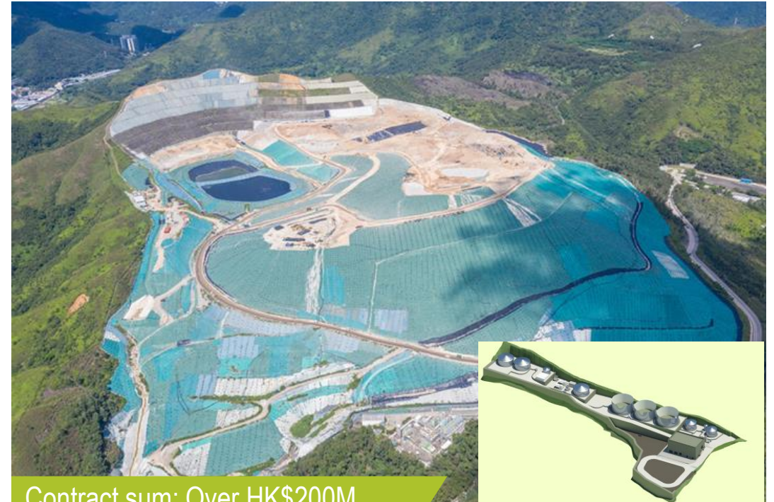
New Leachate Treatment Plant for North East New Territories Landfill Extension (NENTX)
