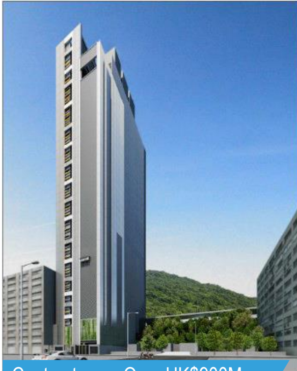
Construction of Government Data Centre Complex
