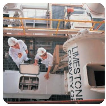
Reducing emissions is an ongoing project of Hongkong Electric. Here the desulphurisation plant "scrubs" sulphur, which reduces emissions.
