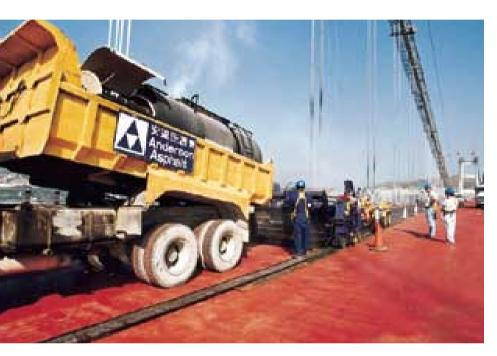
Mastic asphalt was laid on the deck of the Tsing Ma Bridge in Hong Kong.
