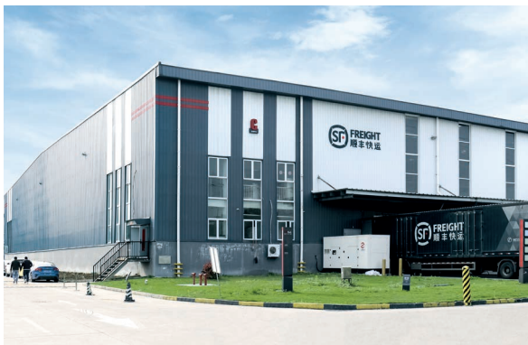
Wuhu Fengtai Industrial Park
