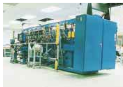
The highly automatic cell assembly line in the Taiwan Lithium Ion battery plant.
