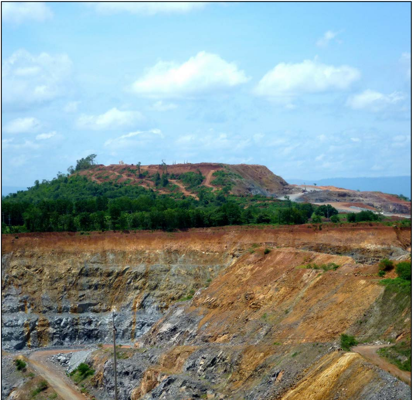
C North cut-back at Chatree with Chatree North A Hill and A Pit in the background.
