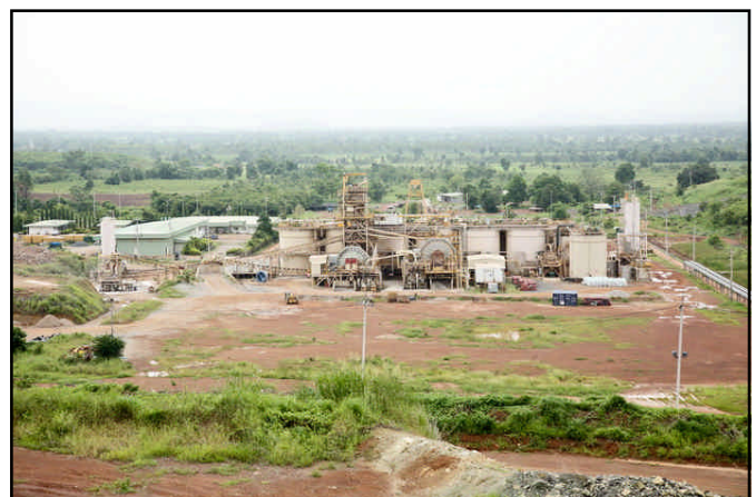
Chatree Plant with area for expanded plant in foreground
