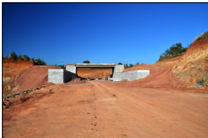
The highway underpass nearing completion north of C North Pit
