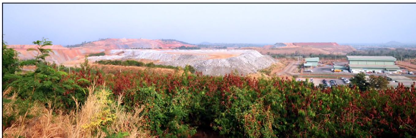
K East Pit being closed (at left), A Hill (in background), stockpiles (in foreground) and new Lotus Hall maintenance buildings at Chatree North (at right)
