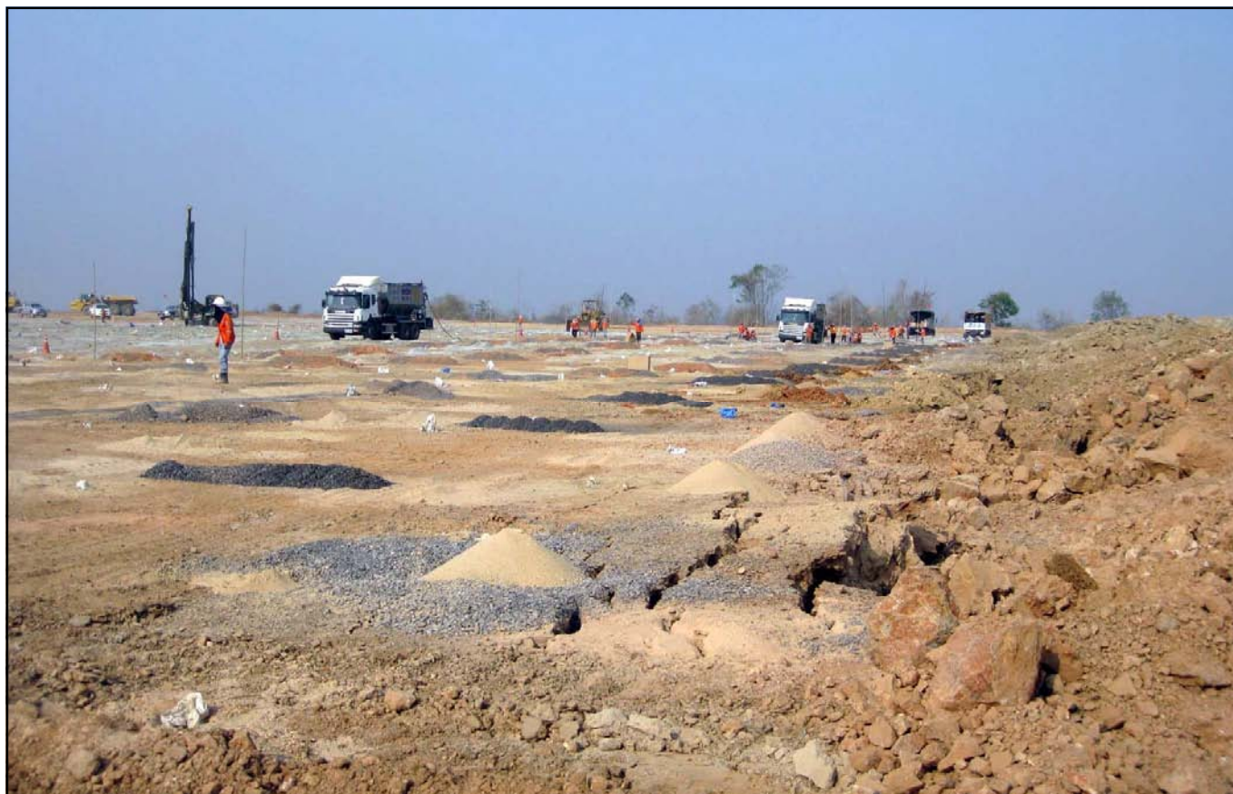
Loading of blast holes on A Hill
