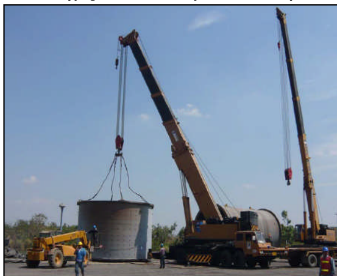
The Ball Mill Heads and both Mill Shells are now on-site.
