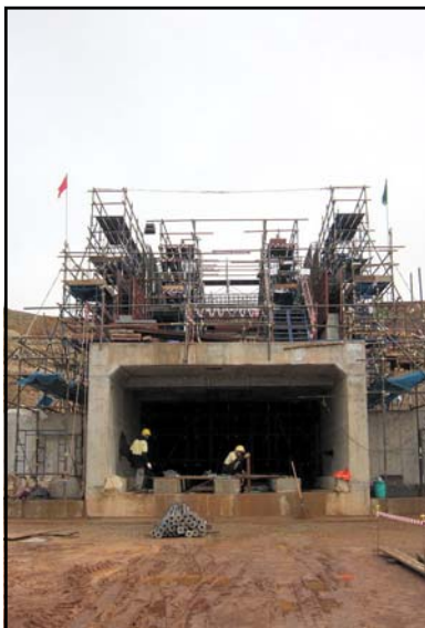
Primary Crusher No 2 under construction
