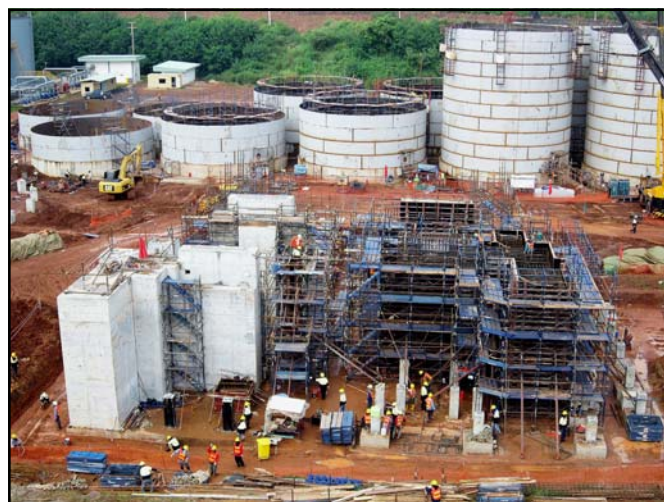
CIP and Grinding Plant (No 2) under construction
