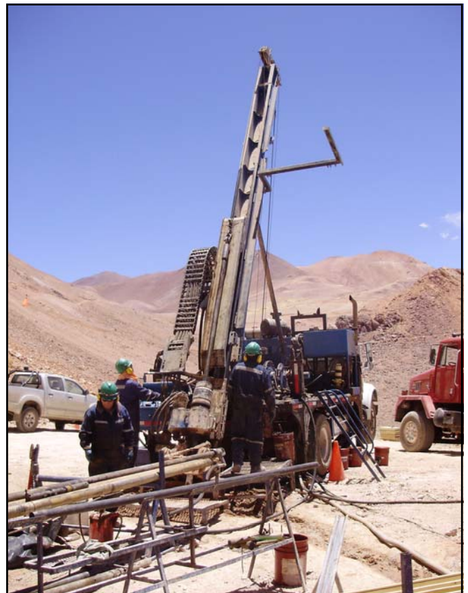
Drilling at the Arqueros Project, Chile.
