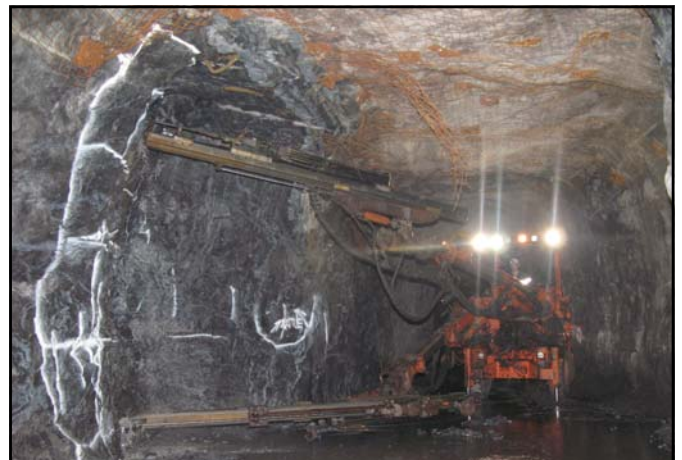
Drilling an underground face at the Challenger gold mine, SA.
