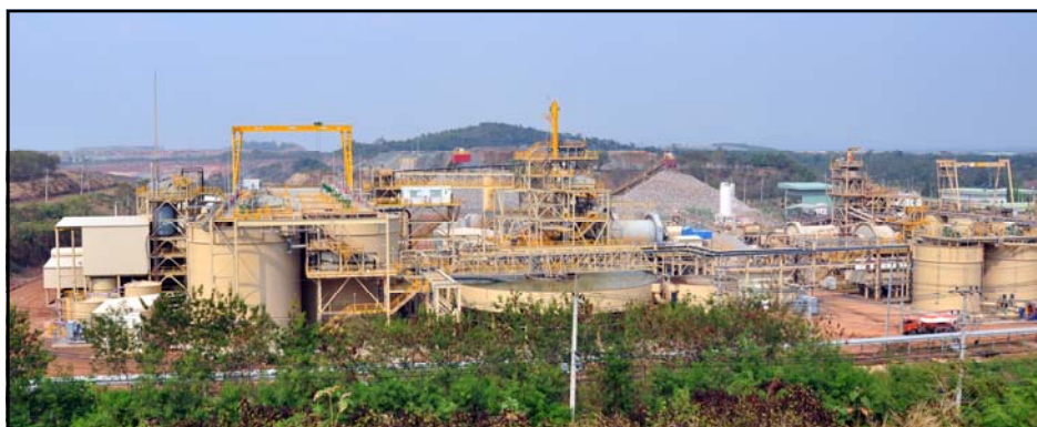
The completed Chatree Expansion Plant.
