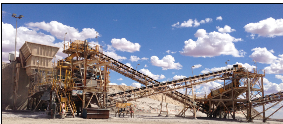
Challenger crushing facilities
