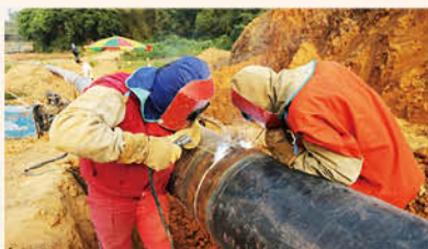
Pipeline welding
